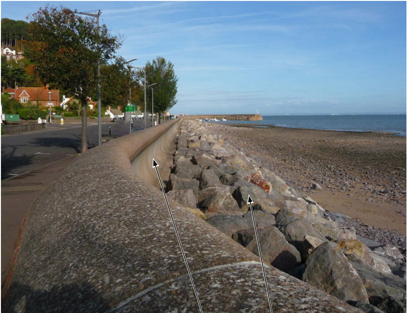
Sea wall and rock armour
